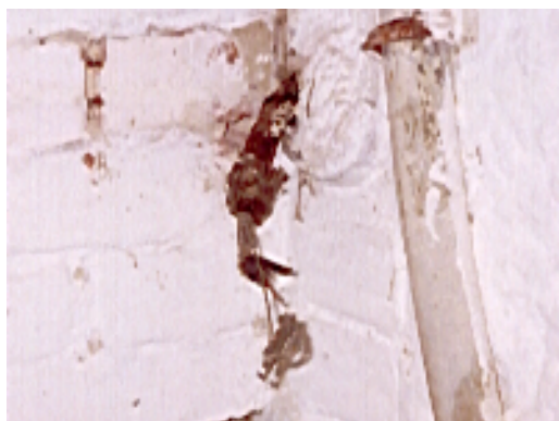
Figure 25 - Old cable entering building
